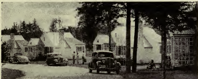
Lakewood Inn: A Street of Bungalows
