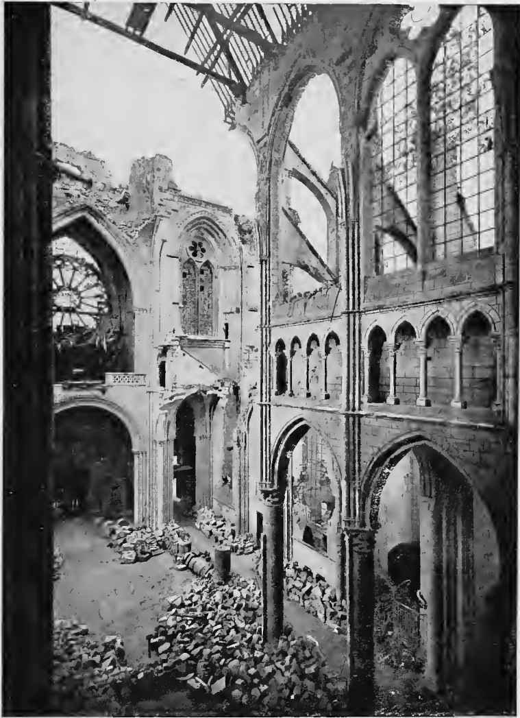
BREACH IN THE NAVE, NOVEMBER 1918
