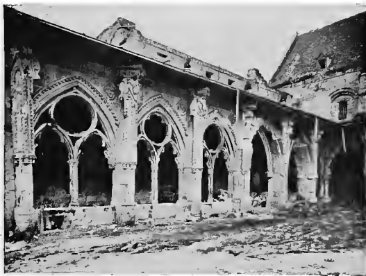
SOUTHERN GALLERY OF THE CLOISTER, NOV. 1918.
