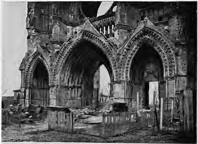
THE DOORWAYS IN THE MAIN FRONT (1918). Part of the ornamental stone-work was damaged by fire in 1870. Keystones of the vaulting were shattered by shell-fire in 1914.
