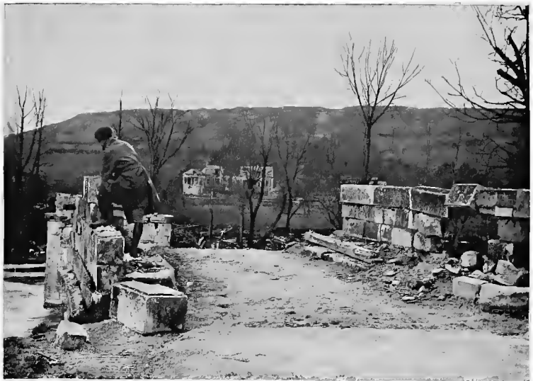
DESTROYED BRIDGE OVER THE AISNE.
