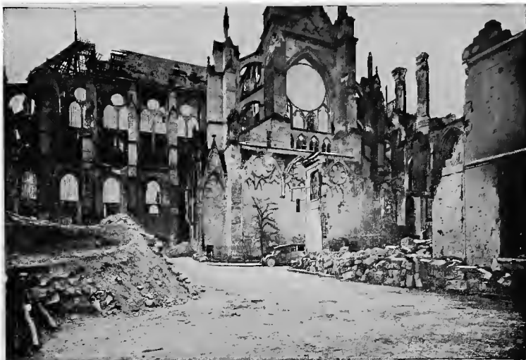
NORTH FRONT. Choir and North Arm of Transept, Nov. 1918. See description, p. 29.
