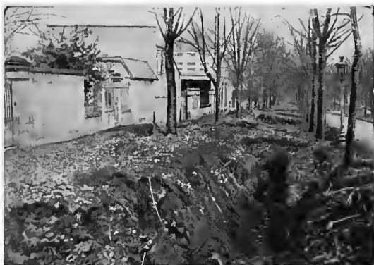
TRENCH IN THE BOULEVARD JEANNE-D'ARC
