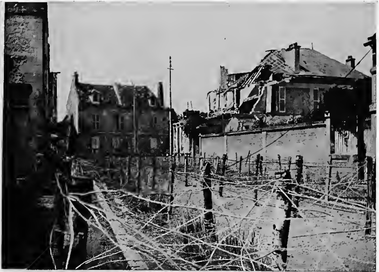
STREET DEFENCE-WORKS IN THE FAUBOURG ST-WAAST.
