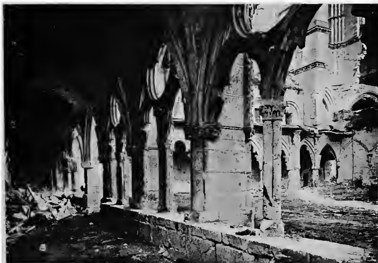
INTERIOR OF THE SOUTHERN GALLERY, NOV. 1918.
