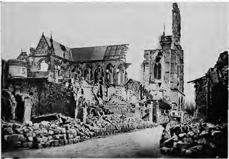
NORTH FRONT. North Arm of Transept, Nave and Chapelle des Œuvres, Nov. 1918.
