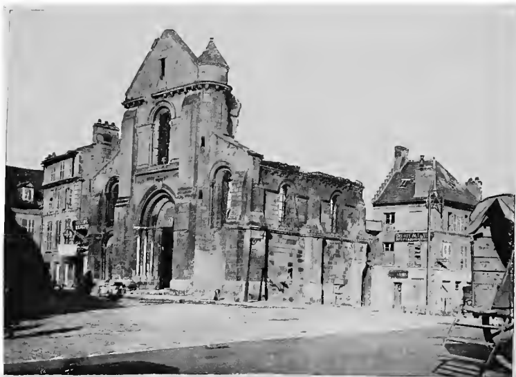
CHURCH OF SAINT-PIERRE- AU-PARVIS. November, 1918.
