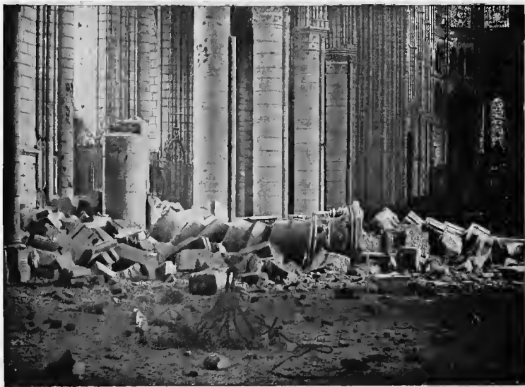
COLLAPSE OF THE PILLAR. FEBRUARY 1915.
