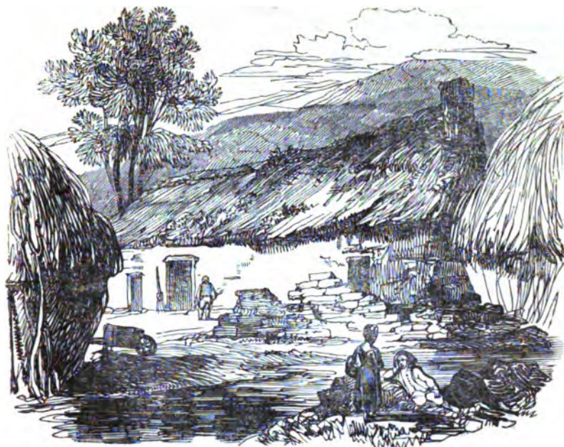
MUIRHOUSE, EAGLESHAM, RENFREWSHIRE.
