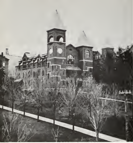
In 1900, Alumni Hall was about fifteen years old. Not only the Normal School auditorium, but also classrooms for the Normal School and Training School were located here.
