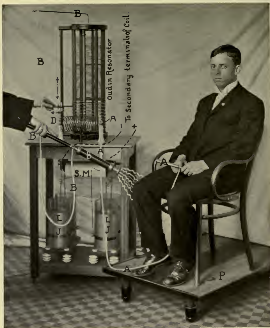
FIG. 67.—Treatment by the effluvia method. The condenser electrode, B , is in connection with the top of the resonator. Patient is seated upon an insulated platform, holding the electrode, A , which is the other pole, from the outer side of the Leyden jar, L J . (By grounding the outer side of the Leyden jar, A , the patient's insulation is unnecessary and better effluvia is attained.) S. M. is the spark-gap.
